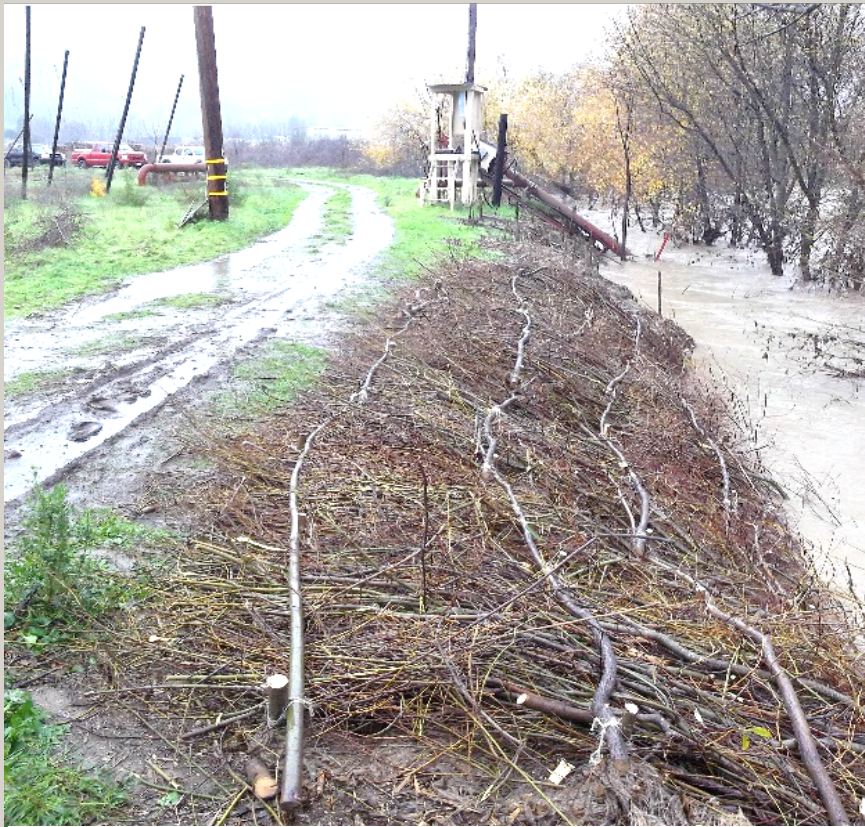
Brush mattress installed in 2016
